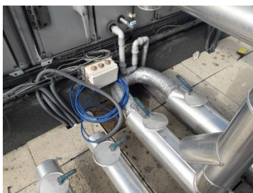
Figure 1 – End of Line Bypass in existing HVAC system.
